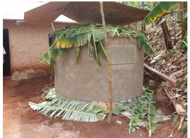
Curing a newly built water tank with banana leaves in Uganda. CWS/ J Gould
